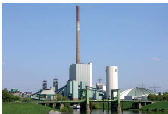
Utility & District Heating
